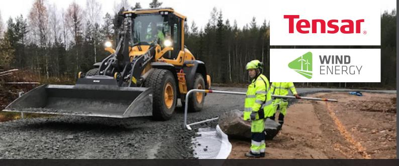
$TriAx\ geogrid\ was\ incorporated\ into\ the\ aggregate\ used\ for\ the\ wind\ farm\ access\ roads\ and\ working\ platforms.$
