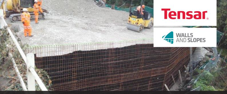
Tensar's TensarTech TR2 system comprised steel mesh face panel securely connected to uniaxial geogrids to reinforce the site-won fill behind.
