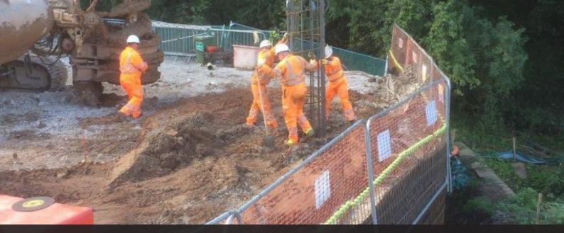
Tensar's TensarTech TR2 temporary reinforced soil wall system delivered a stable, low-cost solution that supported the rig loading of 150kPa, while being quick to build.
