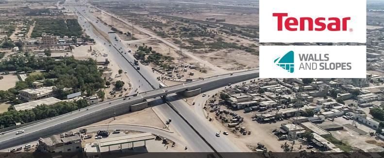
TensarTech® TW1-ME Wall System does not require heavy lifting equipment, minimising disruption to road users
