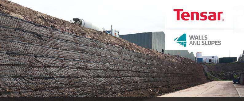
Tensar's TensarTech GreenSlope reinforced soil system helped to maximise development space for new warehouses on the sloping site.
