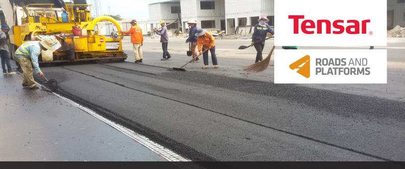
The Stress Absorbing Membrane Interlayer added tensile stiffness, limiting strain and reducing crack development, providing a high performing pavement for the motorcycle circuit.
