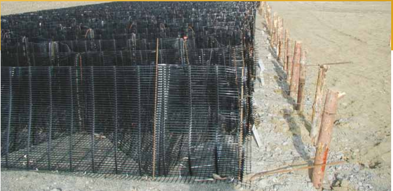
2. Rapid site assembly of the TensarTech® Stratum™ System.
