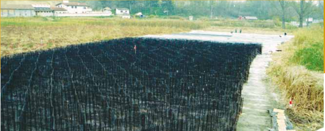
Proven application of the TensorTech® Stratum™ System to stabilise and drain the base of an embankment (Kasposmero, Hungary).
