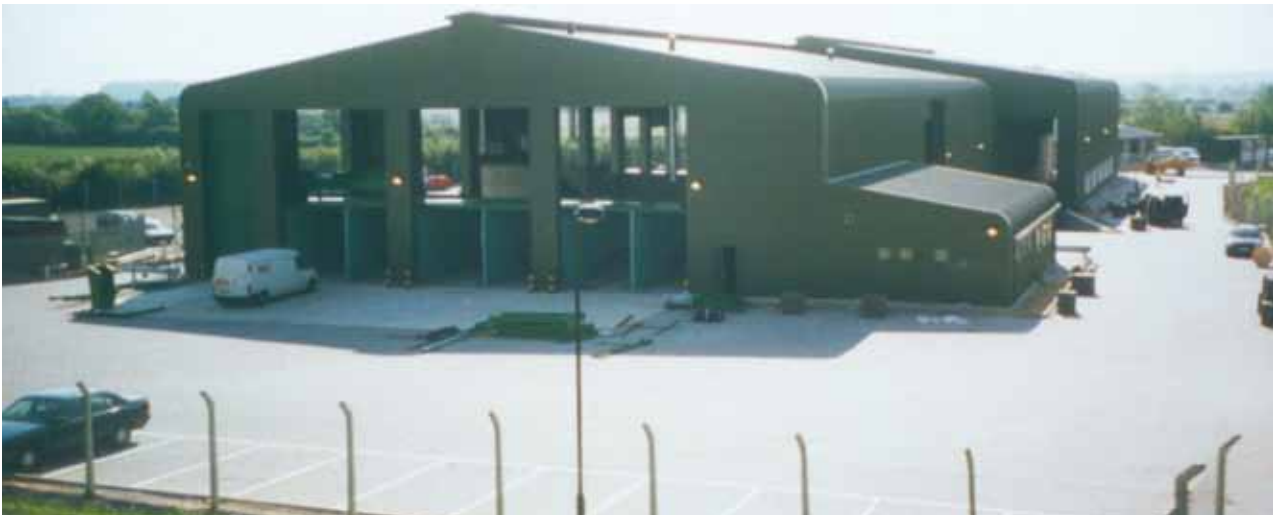
Proven application of the TensorTech® Stratum™ System controlling differential settlement when building over landfill (Elstow, UK).
